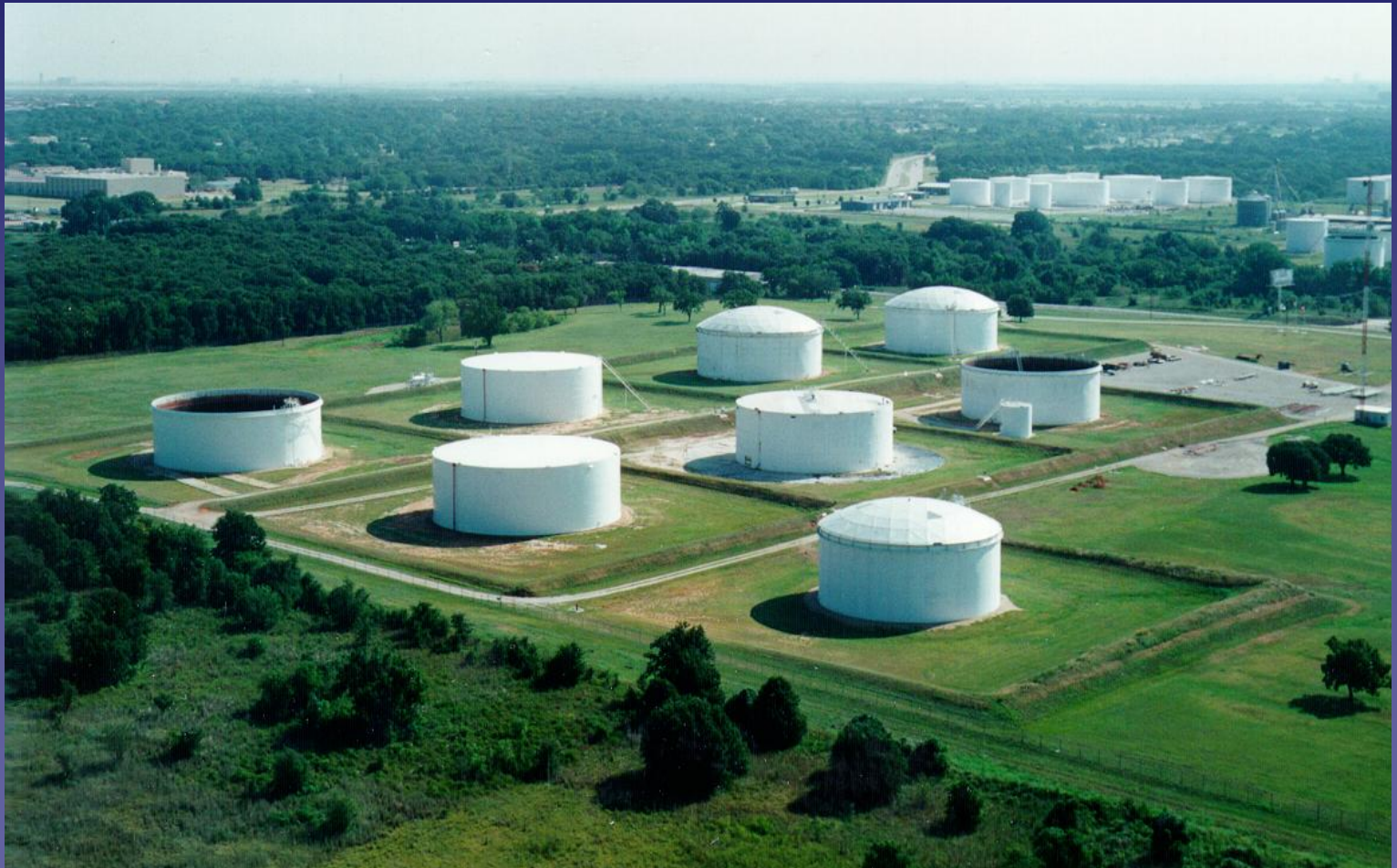
Field Constructed Tanks
