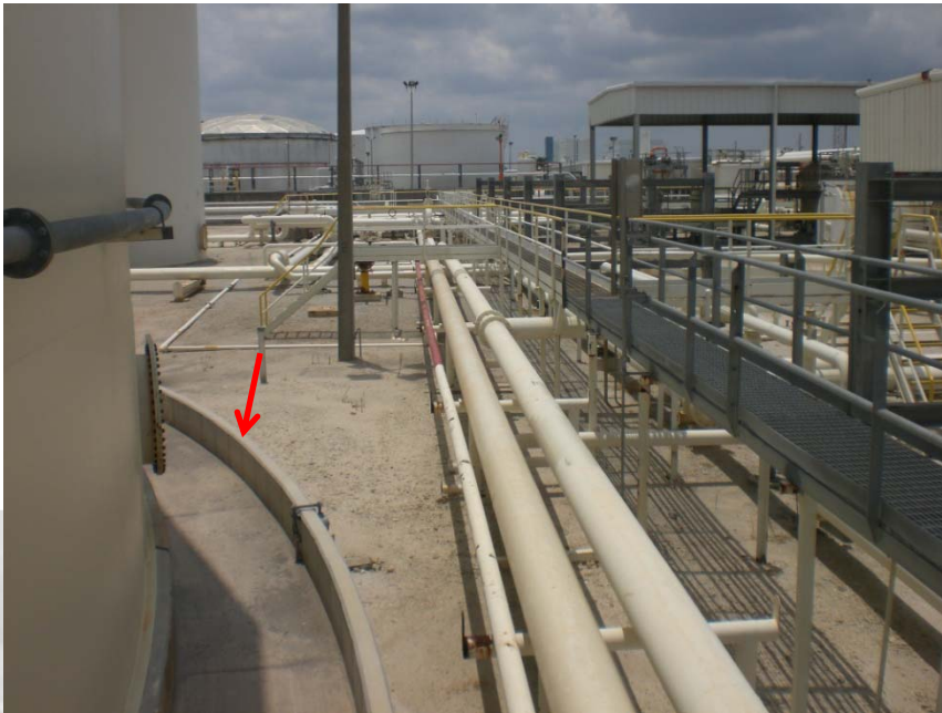
Wall height dictated by tank fill rate
