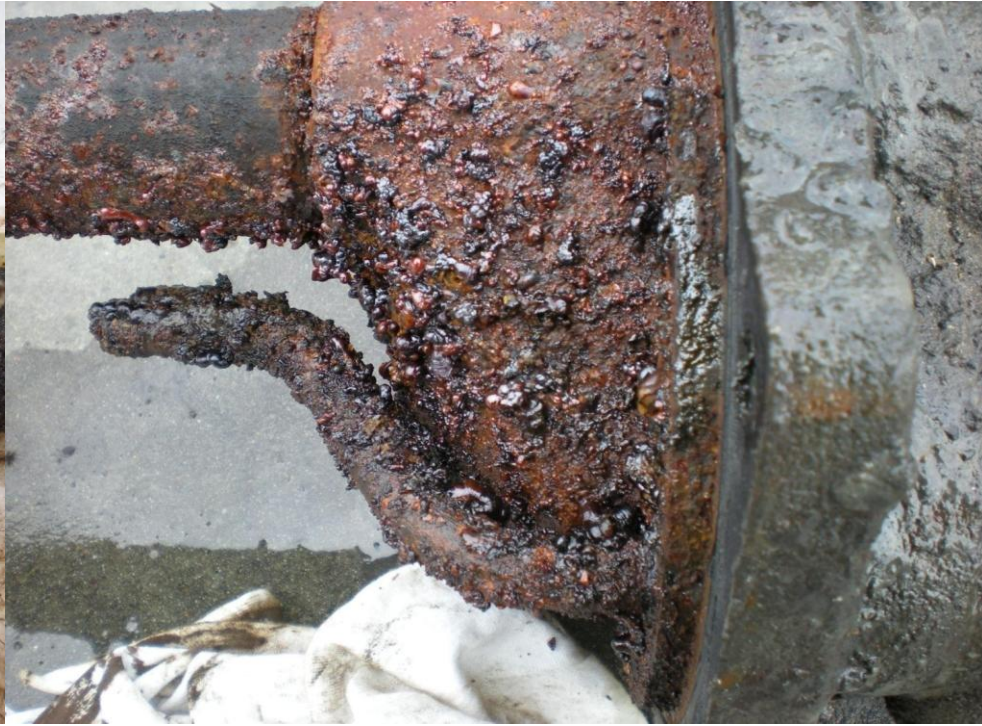
Submersible Pump Head (in vapor space -- never contacts fuel)
