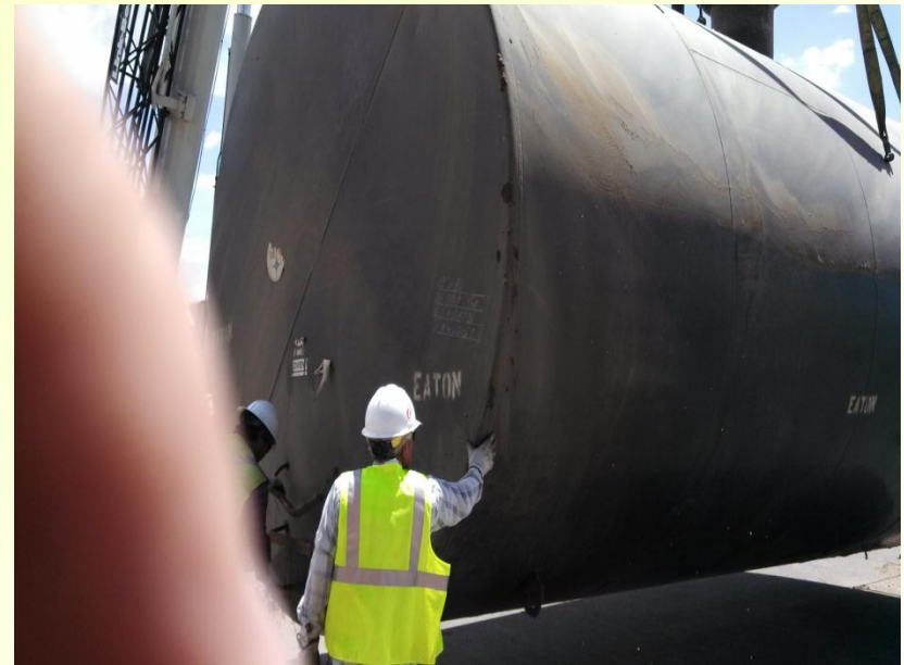
1985 Sti-P3 Tank Removed in 2013 – No Leaks
