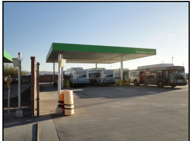
Sky Harbor Bus Refueling Station and Fuel Storage
