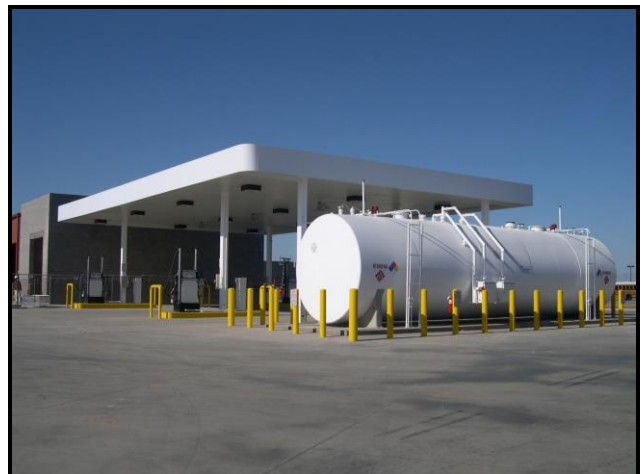
Peoria Unified School District Refueling Facility
