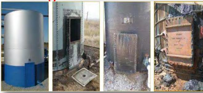
Four tanks with different design specifications, all having rectangular clean out doors.
