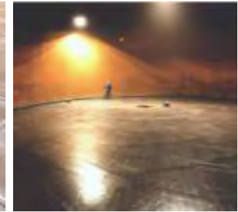
Composite (GRP) One-piece Construction
