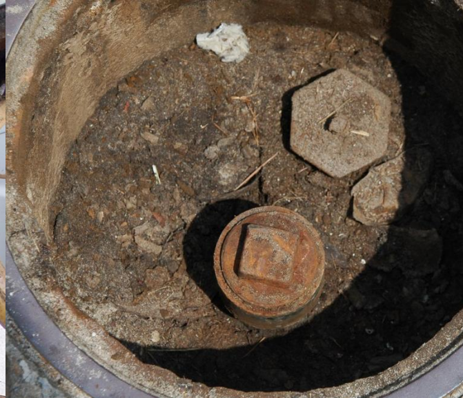
Lubricating and sealing interstitial access ports
