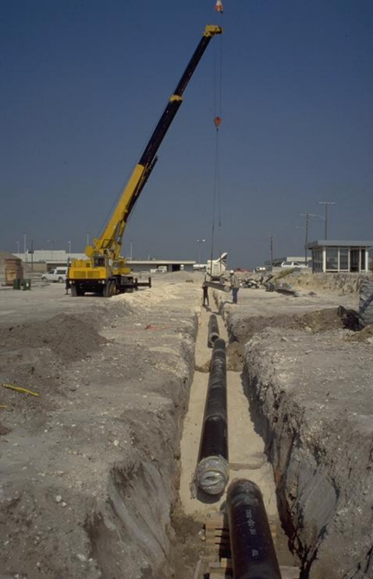
Steel Bulk Product Piping with Secondary Containment - Installation concerns
