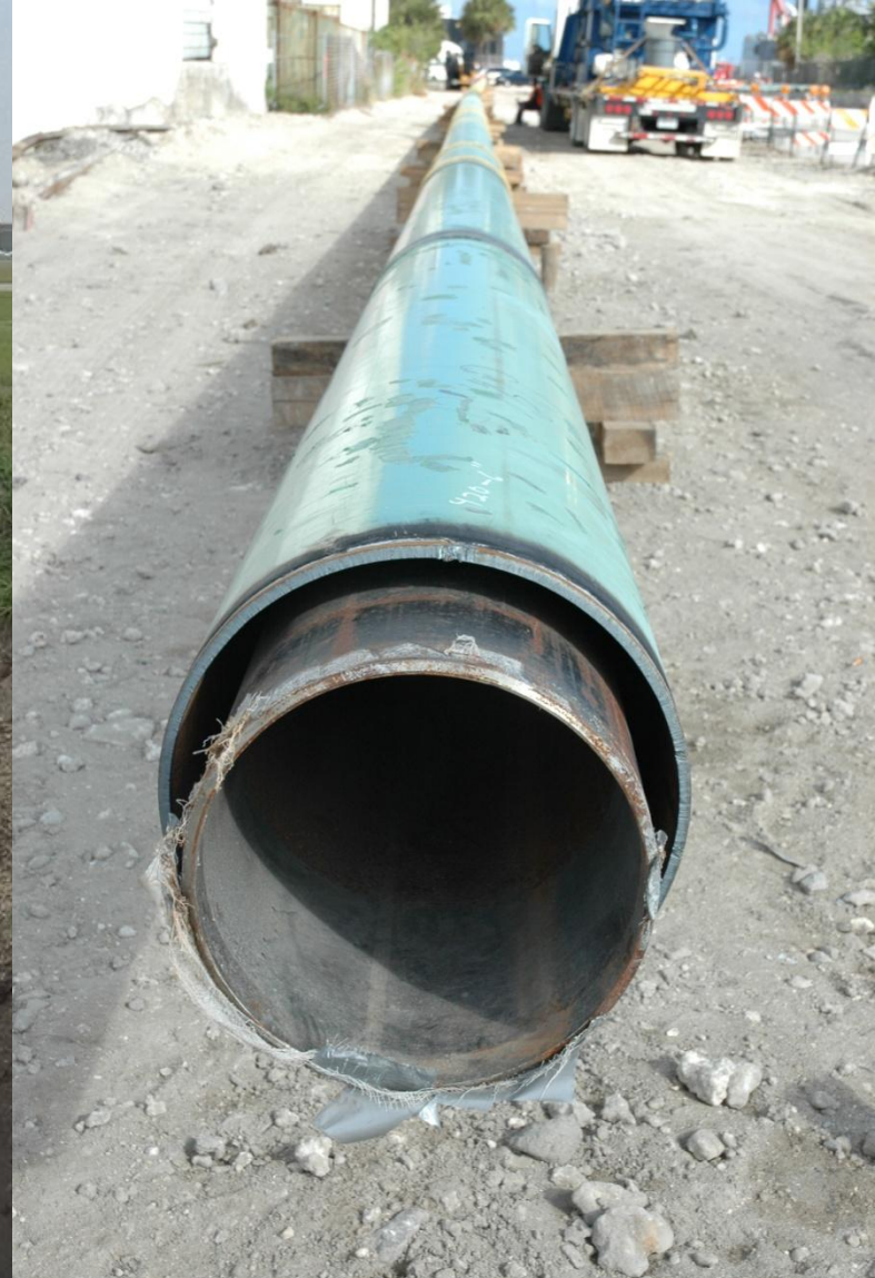
Steel Bulk Product Piping with Secondary Containment - Installation concerns
