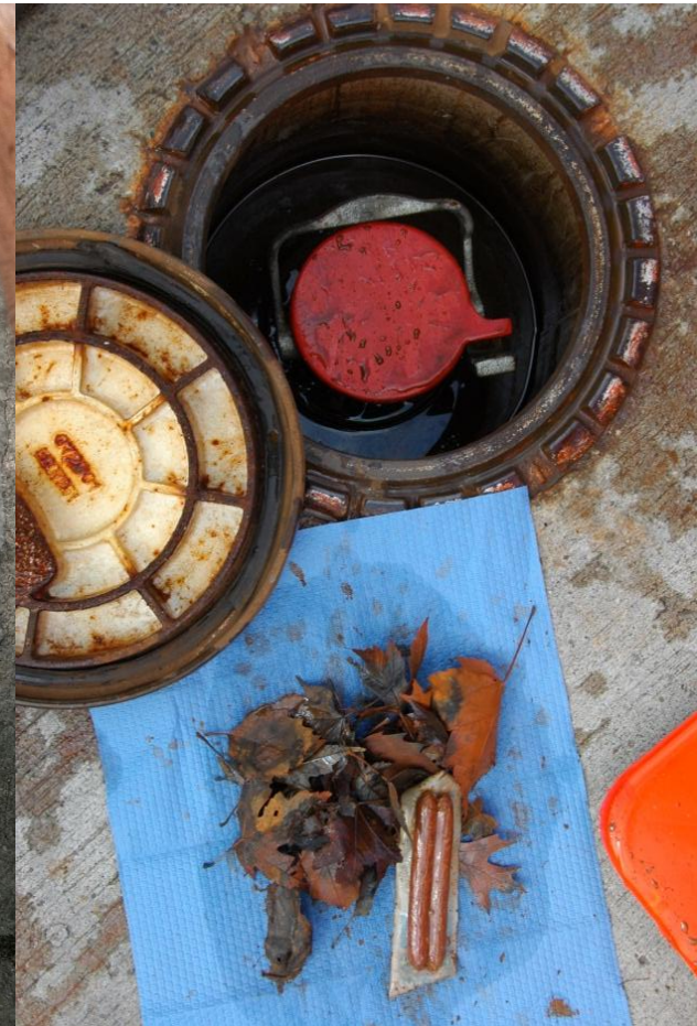
Cleaning debris from sumps
