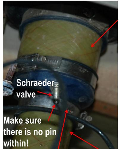
**Outer-wall Piping Leak Detection**
