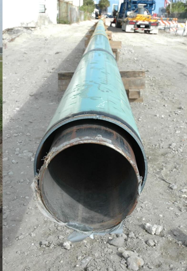
**Steel Bulk Product Piping with Secondary Containment
