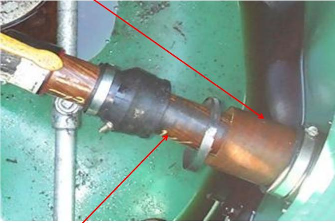
Tight band clamp, no way for product to enter the sump unless the schraeder valve is open
