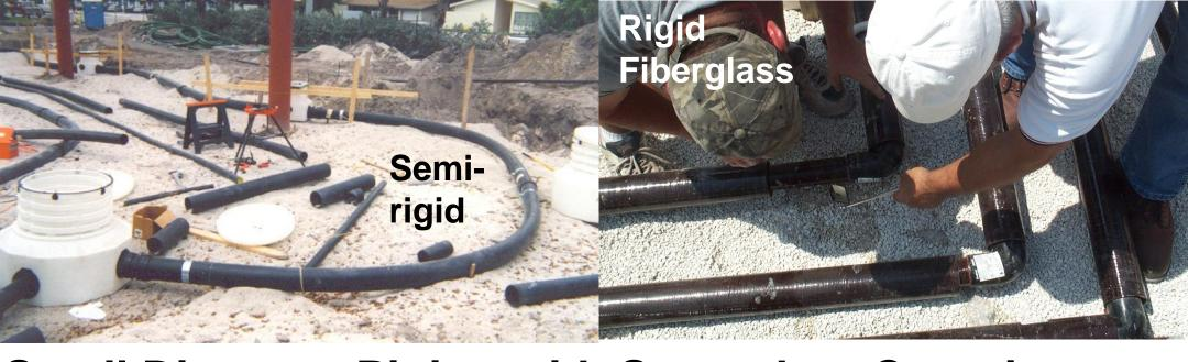
Small Diameter Piping with Secondary Containment
