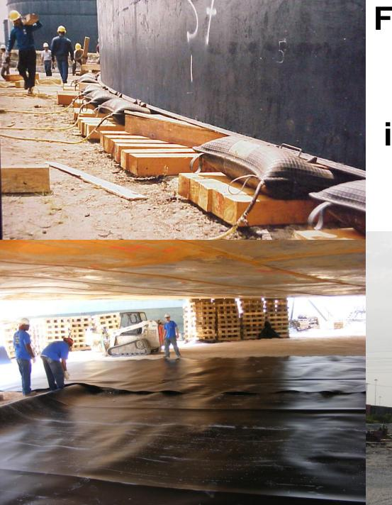
Field-erected AST Lifting for secondary containment installation beneath the tank
