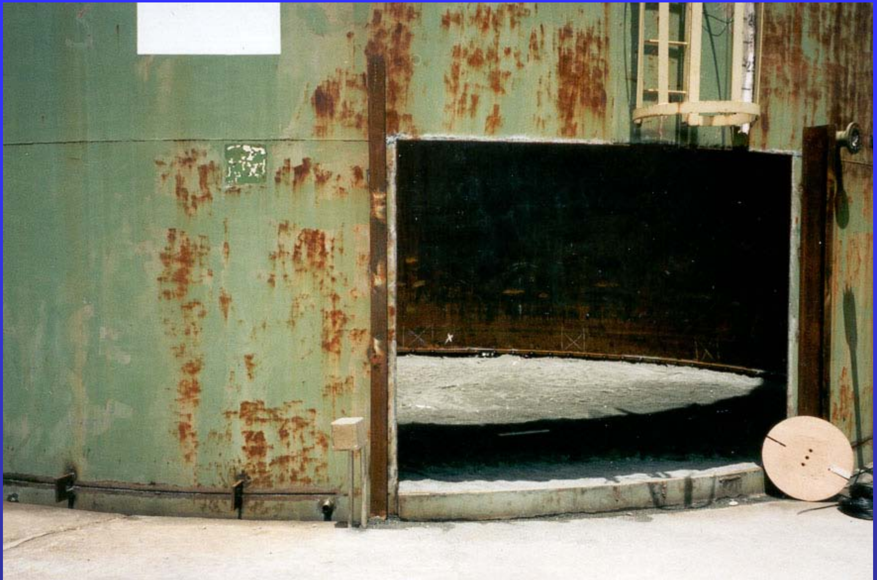
New Floor Installation on Existing AST
