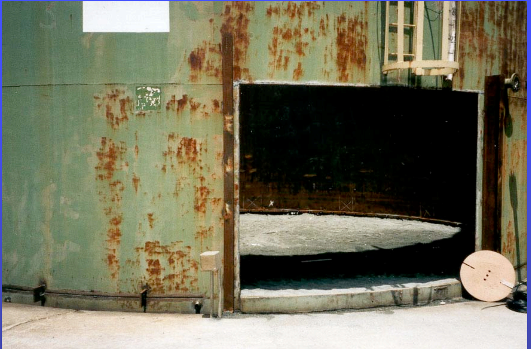
New Floor Installation on Existing AST
