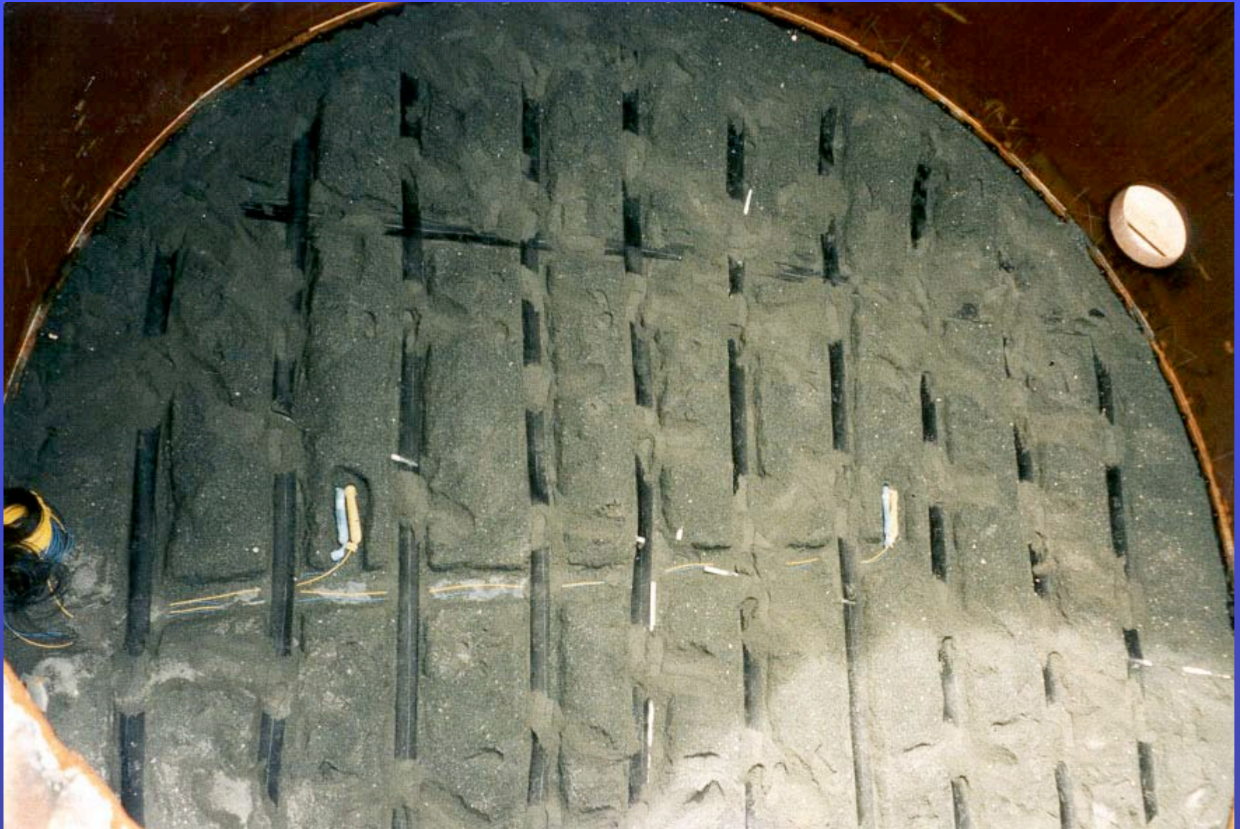
CP Installation on Rebottomed Tank
