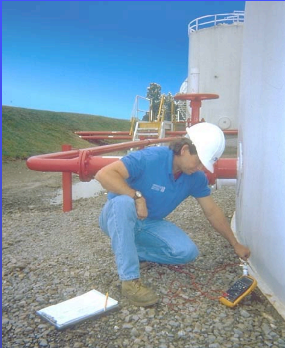
Annual Cathodic Protection Survey
