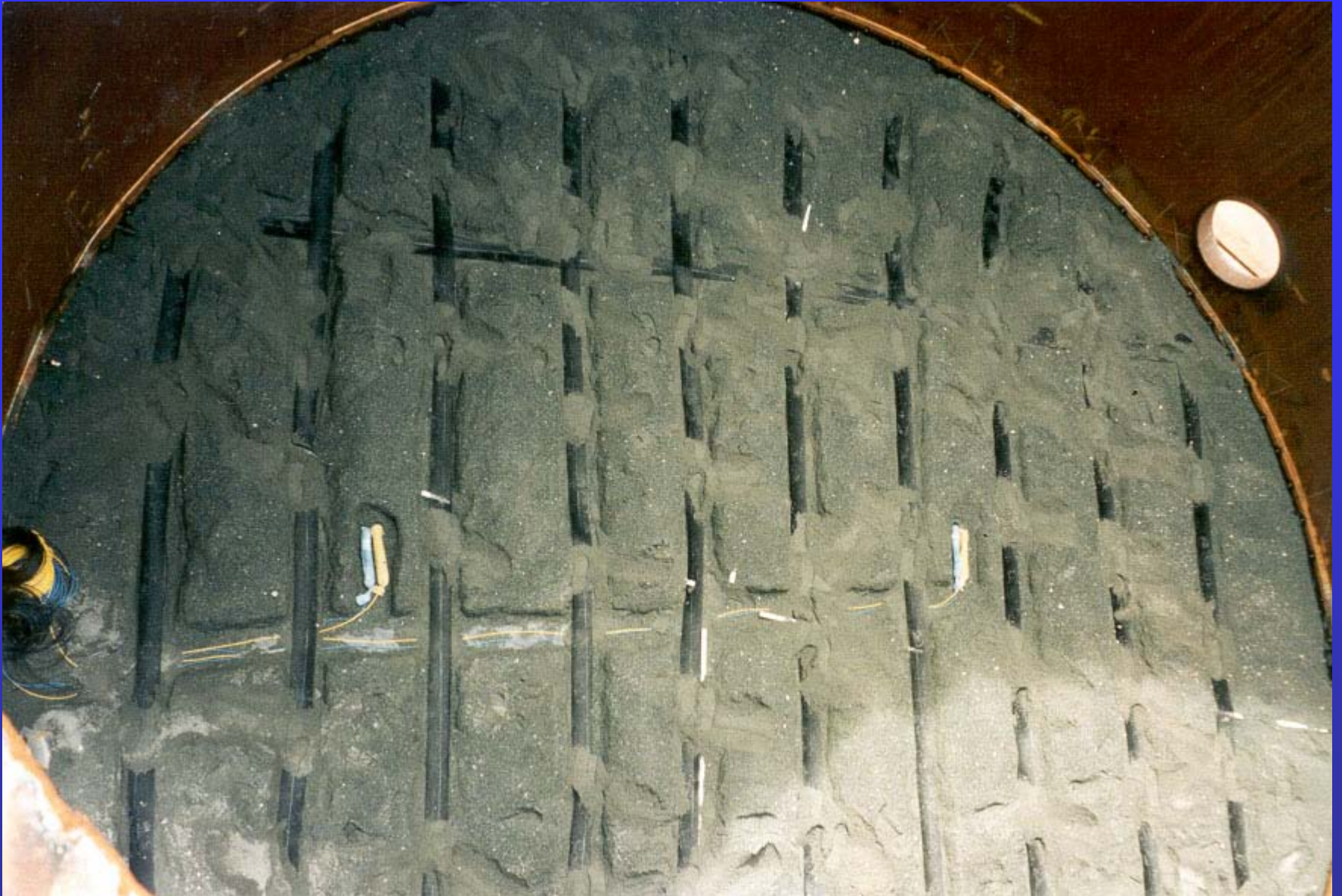
CP Installation on Rebottomed Tank
