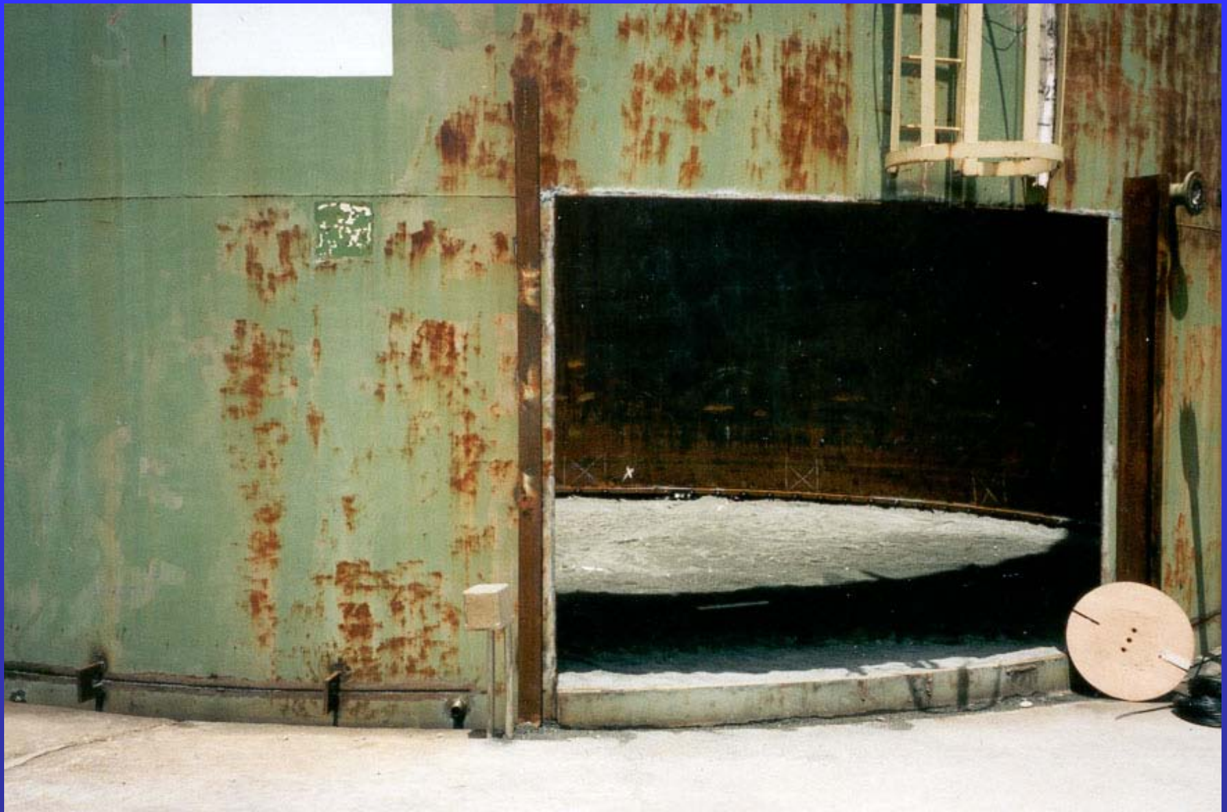
New Floor Installation on Existing AST
