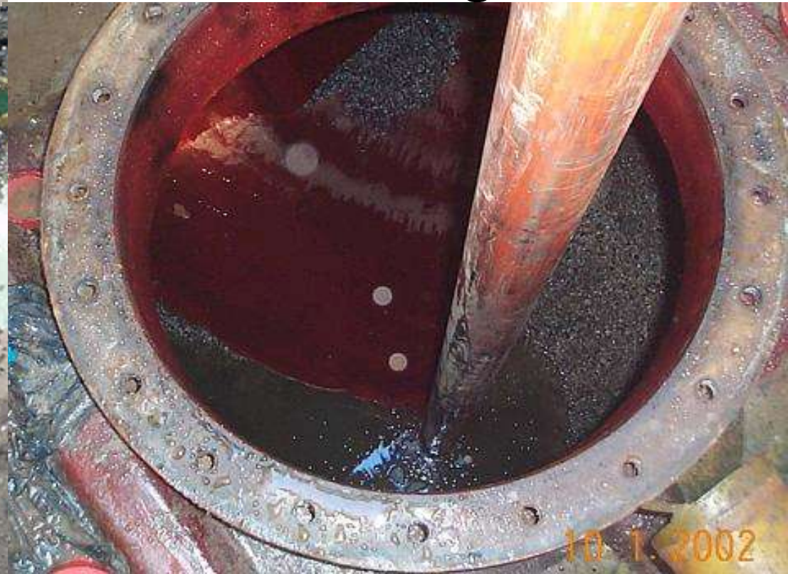
Fiberglass tank void - discharge
